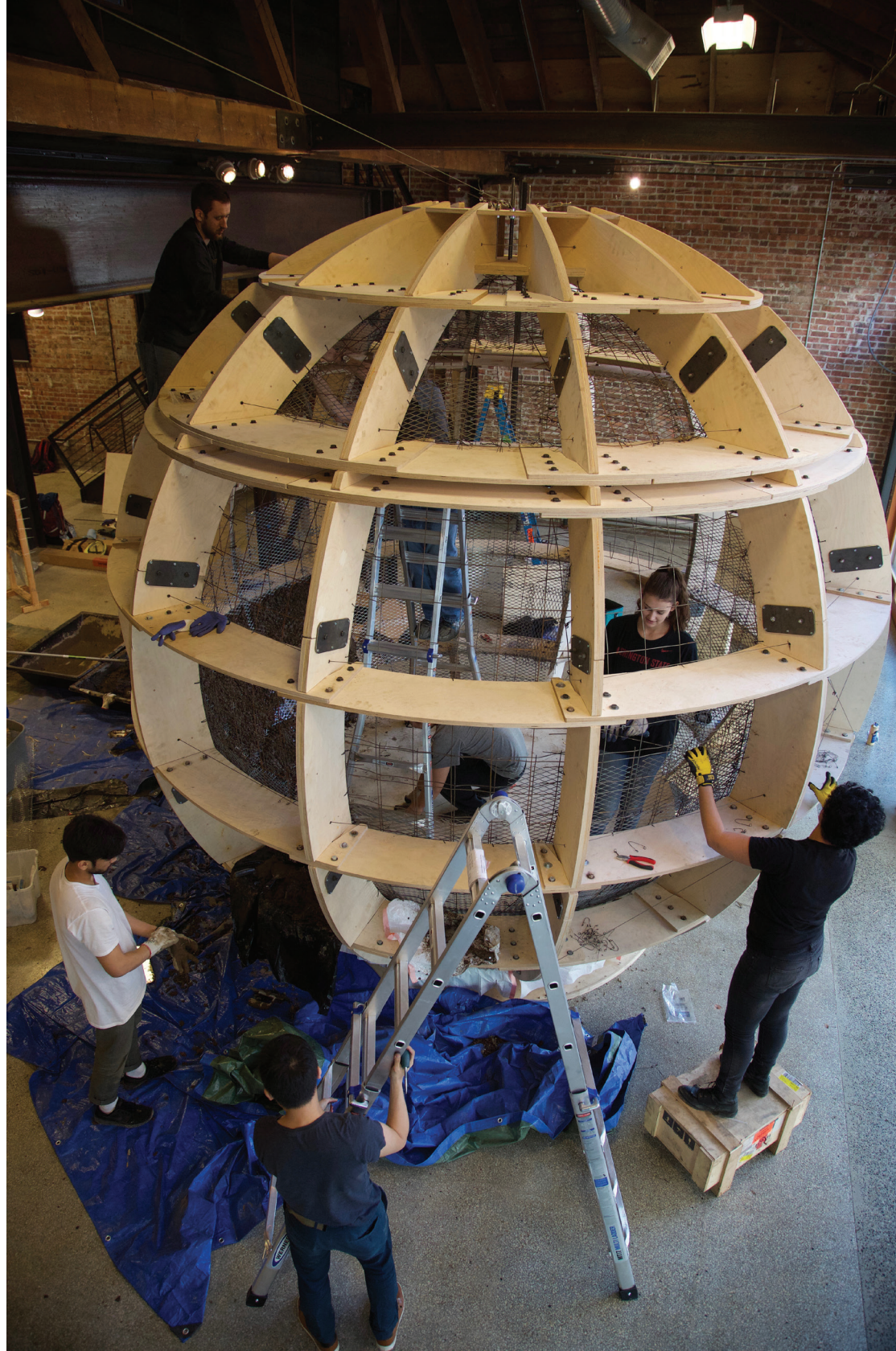
LEFT: WSU ARCHITECTURE GRADUATE STUDENTS AND PROJECT ASSISTANTS WORKING TOGETHER TO CONSTRUCT THE MODULAR FRAME FOR EARTHEN LIGHT
